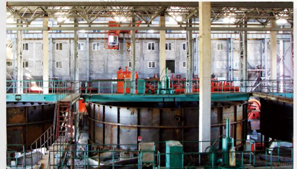
Phosphorite mine with capacity of 1000t/d in Guizhou, China
